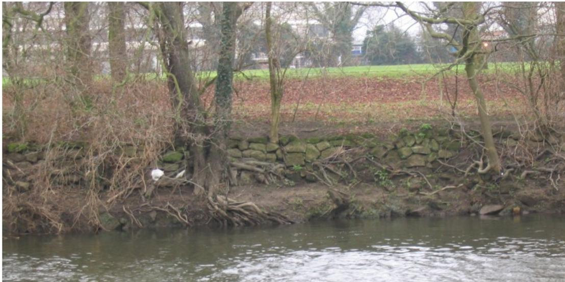
This is the wall that has been exposed due to the scouring effect of the recent floods. Photograph taken 29/01/2008
